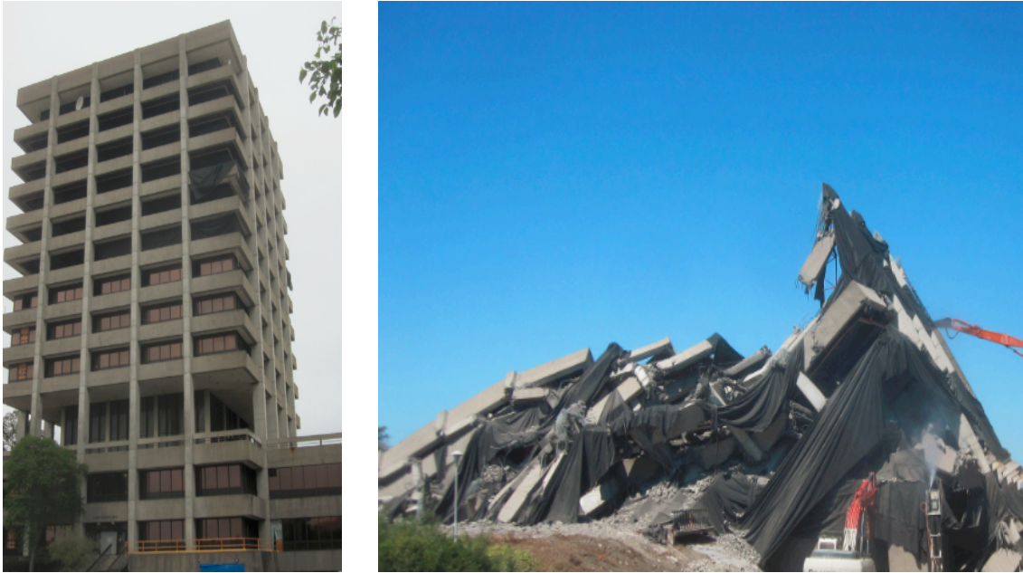
FIGURE 4. WARREN HALL BUILDING – BEFORE AND AFTER IMPLOSION.
